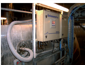
Direct stack installation
