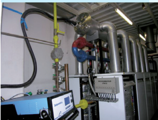
Example: combustion process control using transportable Graphite 52M analyzer
